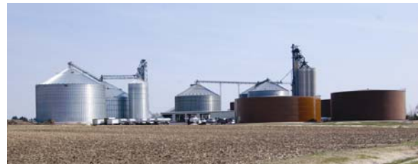
4. The United Cooperative South Beaver Dam location is one of their largest grain locations. It's also the parent location for United Cooperative's agronomy division, including the largest amount of liquid and dry fertilizer storage in Wisconsin. The location and its employees were recognized by DuPont Crop Protection as the 2011 National Environmental Respect Award winner at a special ceremony in the Longworth House Office Building near Capitol Hill in Washington, D.C. on July 14, 2011.
