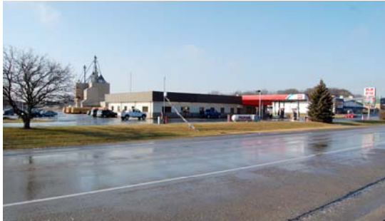
1. The United Cooperative corporate office is located in Beaver Dam, Wis. It's pictured here with United Cooperative's Beaver Dam Cenex convenience store and state-of-the-art Beaver Dam feed mill.
